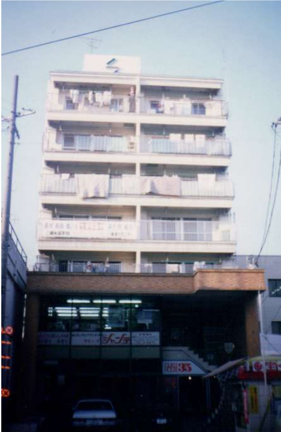
The south side of our apartment building. Our apartment is on the top floor, leftmost unit. If you squint, you can see me standing on the balcony near the centerline. If you squint really hard, you can see Ishida behind the sliding glass door behind me, photo bombing.
